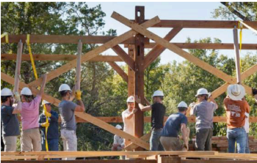
Volunteers building a Micro Home at Community First! Village
