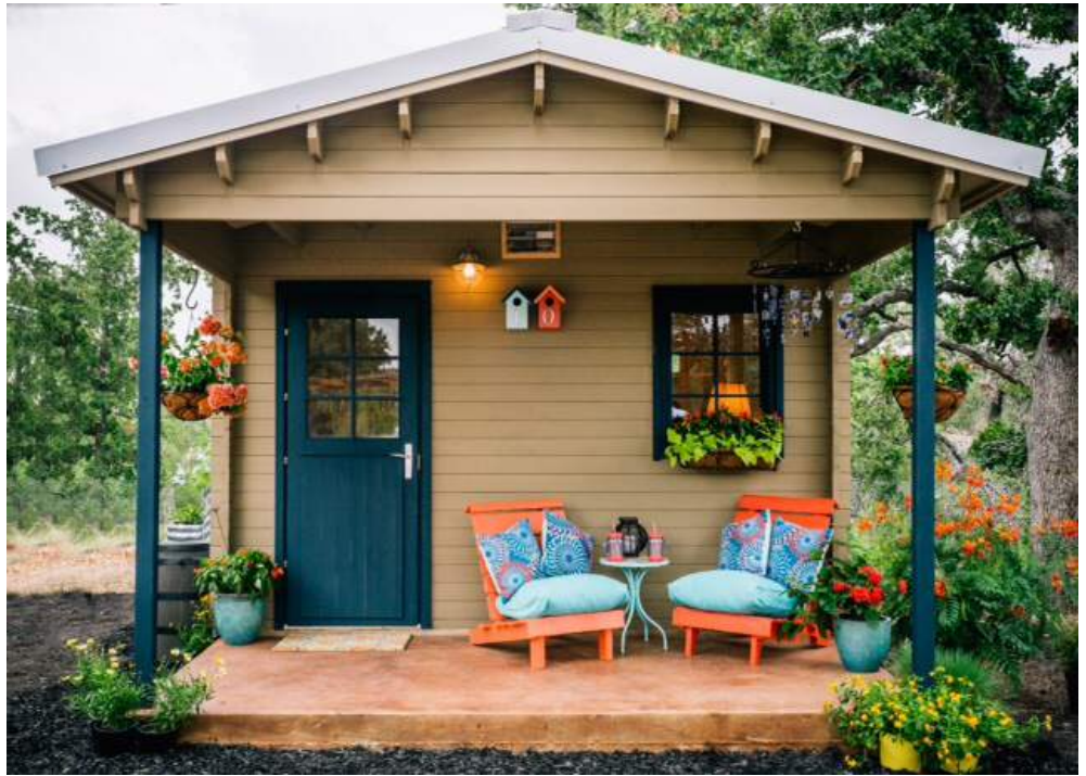
Finished Micro Home at Community First! Village
